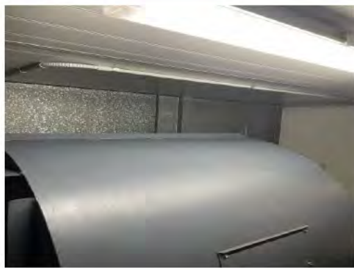
Image 14 – AHU 1.A Supply Air Plenum After
