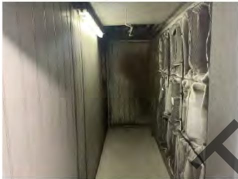
Image 17 – AHU 1.A Return Air Plenum Before
