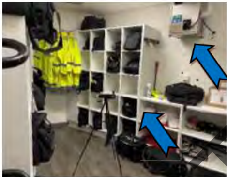
15. CTPI [redacted] Kit Room, CTPI [redacted] - Various timber shelving containing officer contents was observed throughout. Also, a permanently installed dehumidifier was noted to be in operation.
