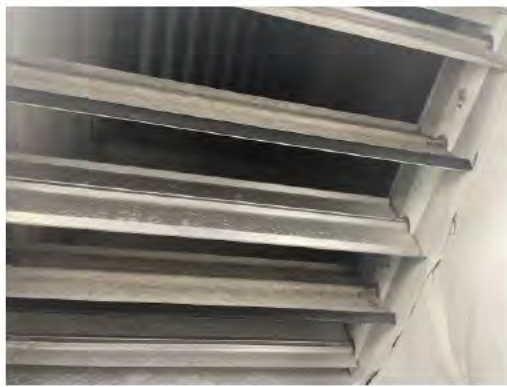
Image 15 – AHU 1.A Return Air Plenum Before
