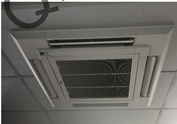
New ceiling cassette in AC-4 zone
