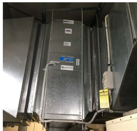
HRW with isolator tagged-out
