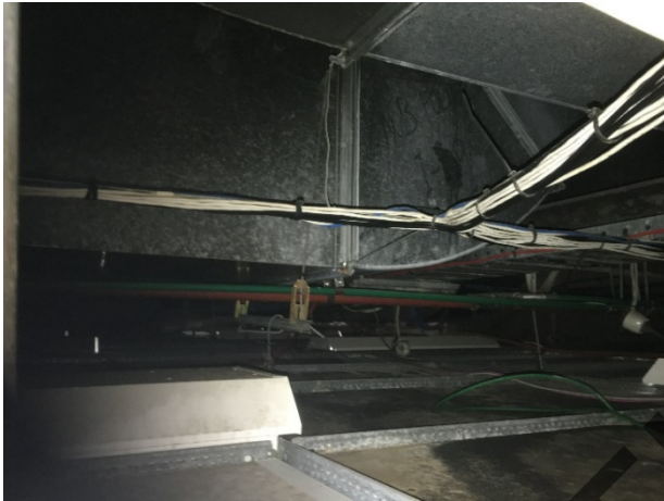
Typical ceiling space
